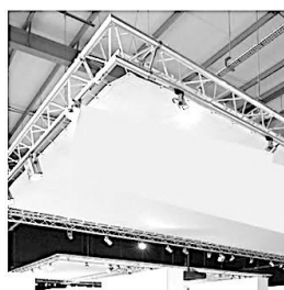
Example of temporary and demountable structures from left to right: totem, self-supporting arch, suspended light bridge with sign
