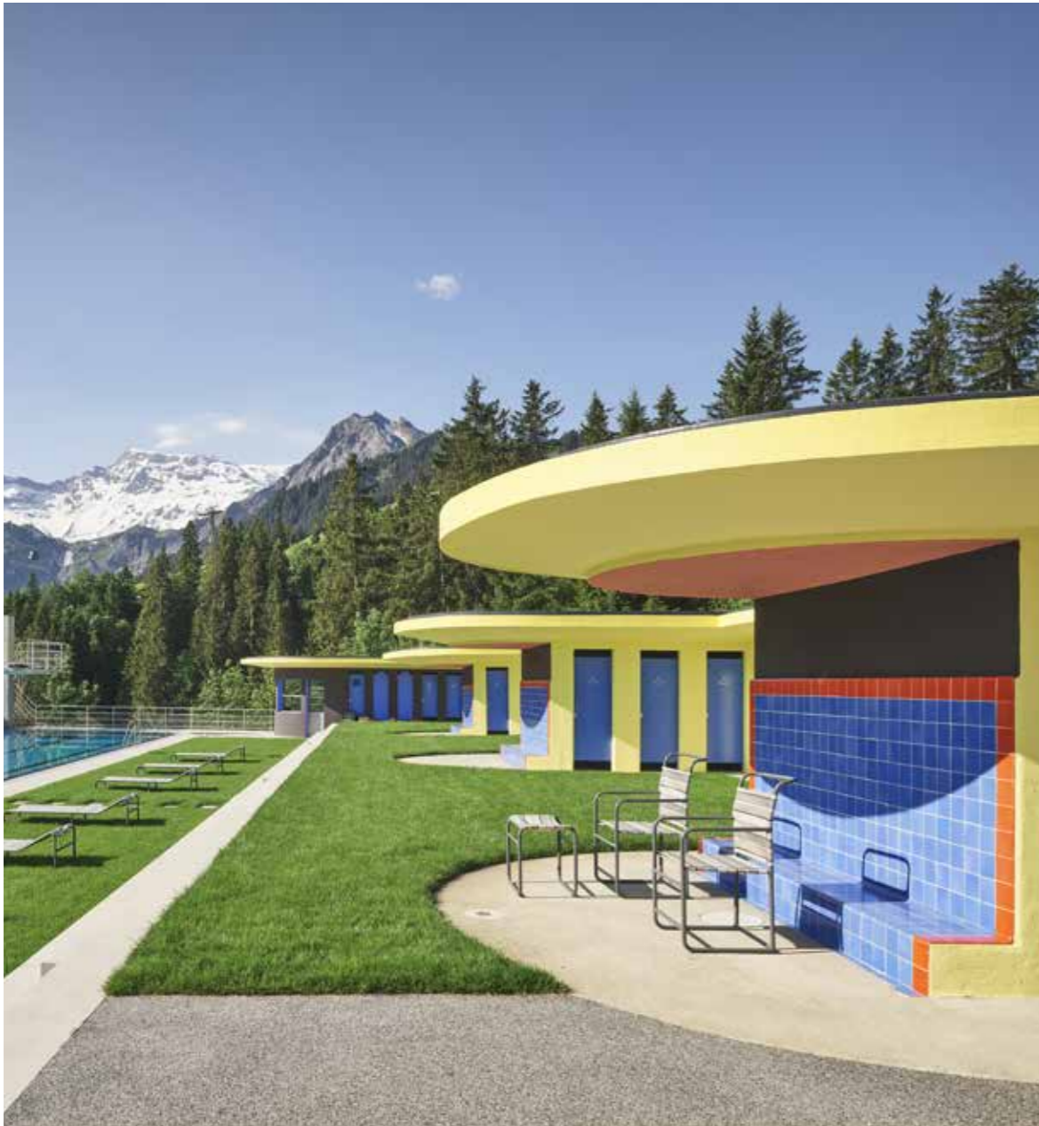
Outdoor Pool Gruebi Adelboden, CH
