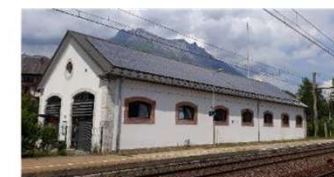
Ateliers des quais 36 kWc – 2023 – Autoconso collective
