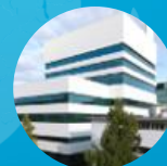
Pharma facility SWITZERLAND
