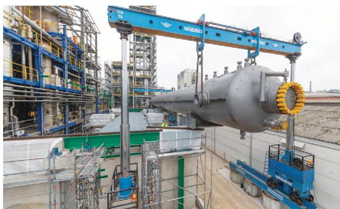
The vertical lift from the low-loader onto the foundations using a hydraulic gantry system.
