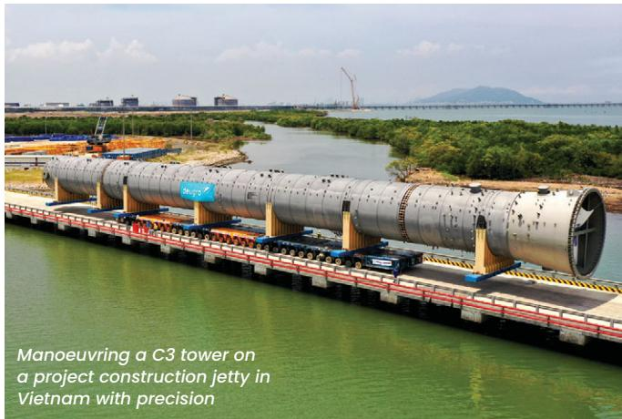
Flexibility and coordination were key to the successful delivery of 280,000 freight tons of petrochemical equipment from over 30 points of origin to a petrochemical plant construction site in Vietnam while Covid restrictions were in force.
