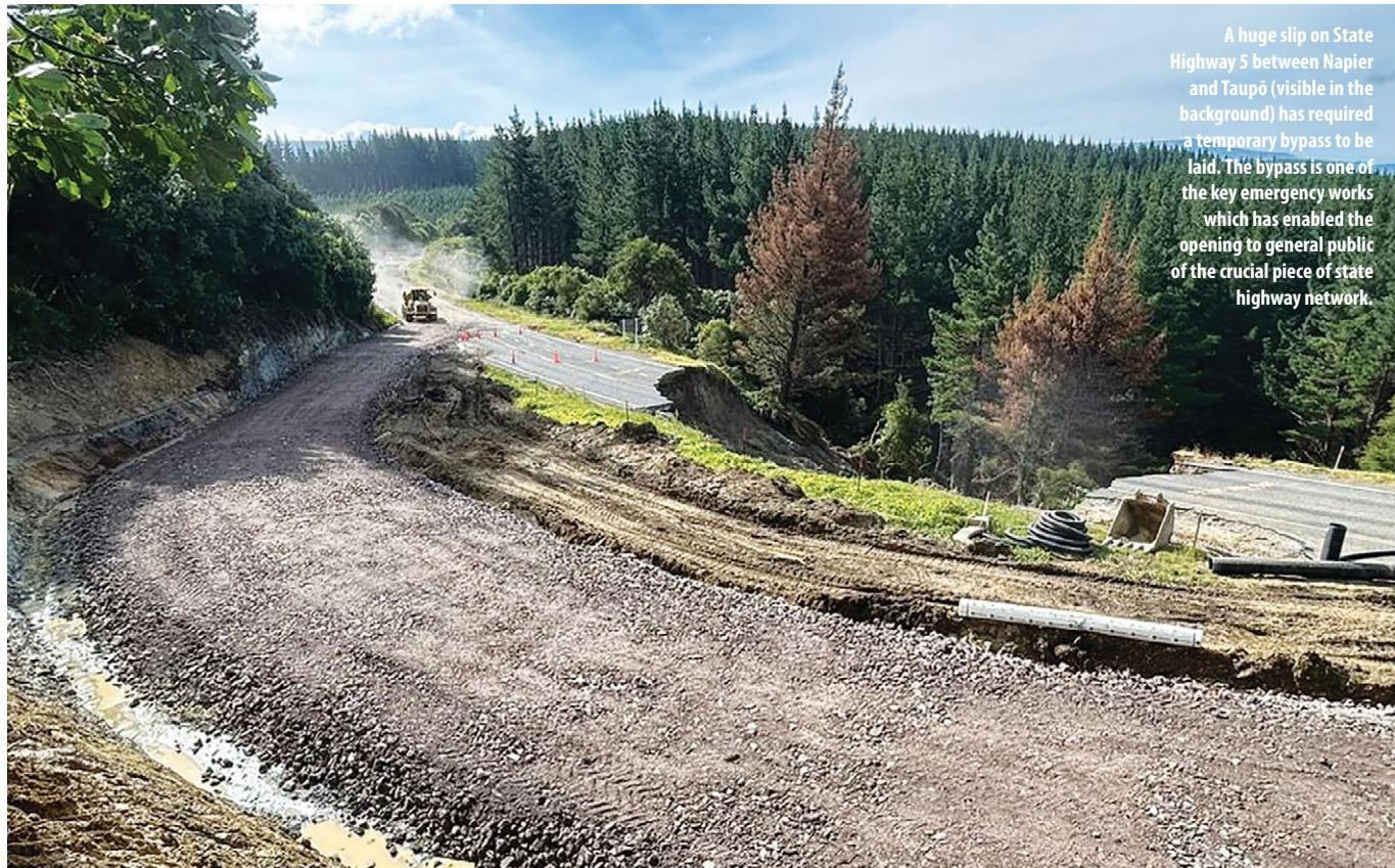
A huge slip on State Highway 5 between Napier and Taupō (visible in the background) has required a temporary bypass to be laid. The bypass is one of the key emergency works which has enabled the opening to general public of the crucial piece of state highway network.
